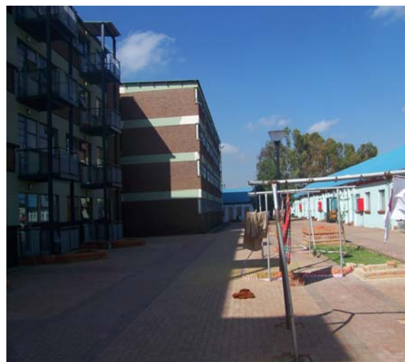
© Benit-Gbaffou, 2009. On the right, the renovated “123 units”; on the left, renovated Block E; at the back, the “Decant Block” where displaced tenants wait for their units to be ready for occupation.
