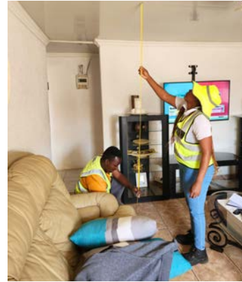
Left: Wattville Sensor Installation Team recording the households building dimensions to understand the households building characteristics.
